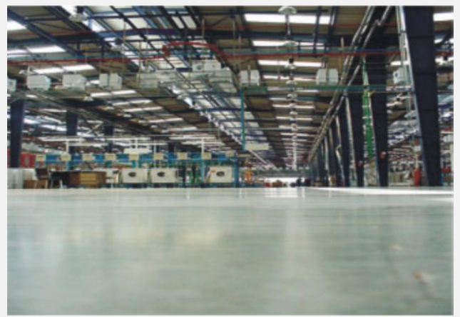
Fig 1: factory floor achieved by Novo Hard Floor
